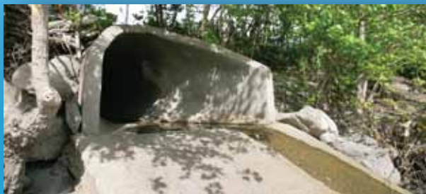
Storm Drain Outfall
