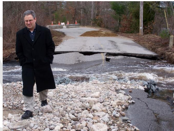
France Street Bridge
