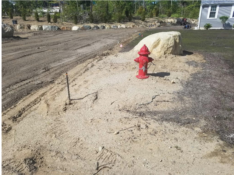
Photo 8: Hydrant where gate valve could not be located
