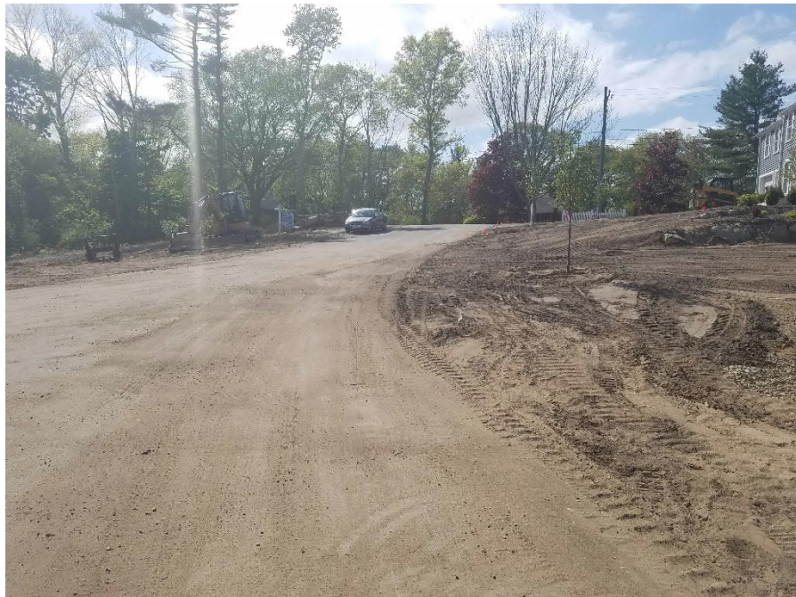
Photo 5: Roadway in front of Lot 2
