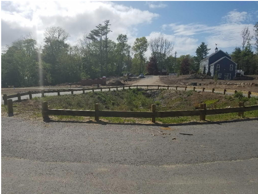
Photo 7: Guard rail and bioretention basin
