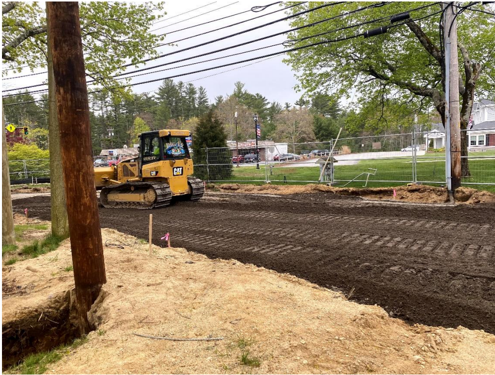
Prepping Road to Subgrade
