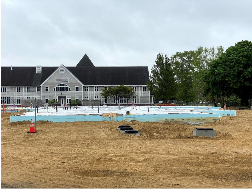
Wet Curing Slab on Grade
