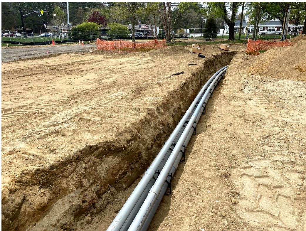
Installation of Telecommunication Lines
