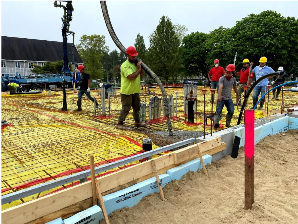
Pouring Slab on Grade
