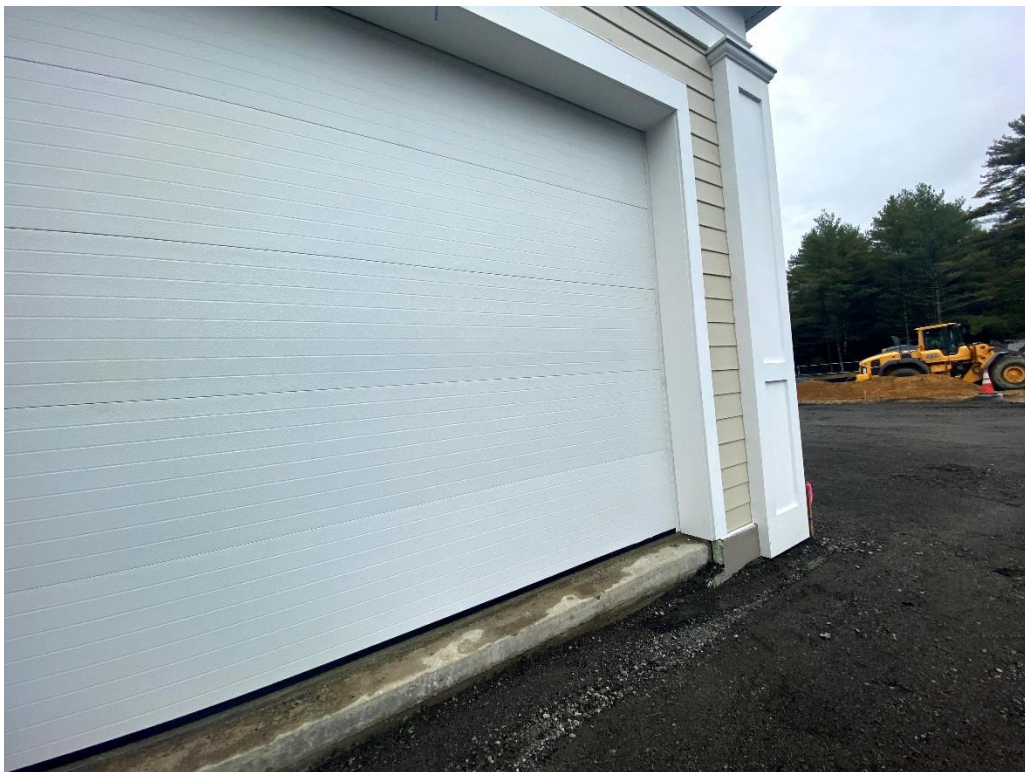
Overhead Door Installed at Sally Port
