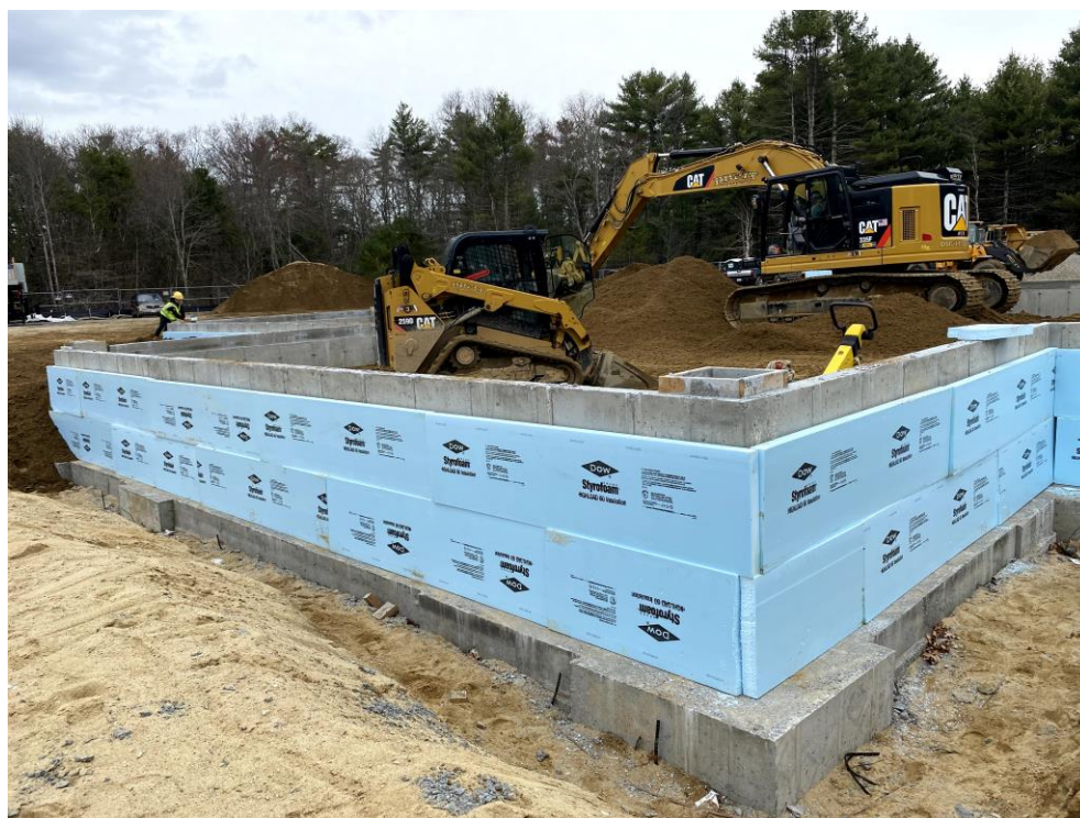
Rigid Insulation Installed
