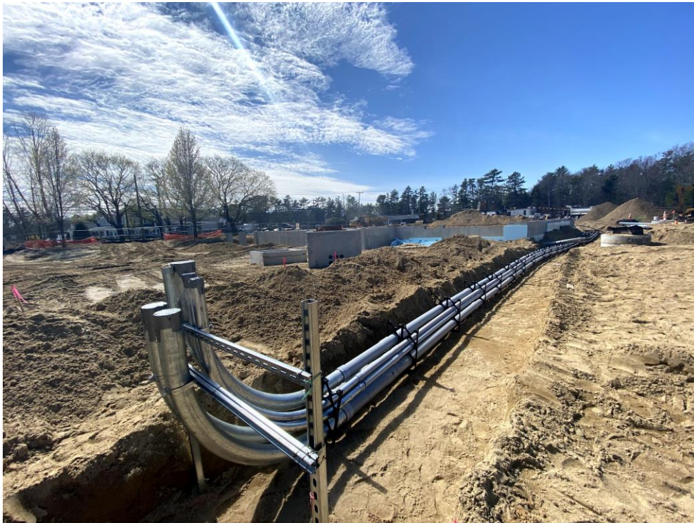
Electrical Ductbank
