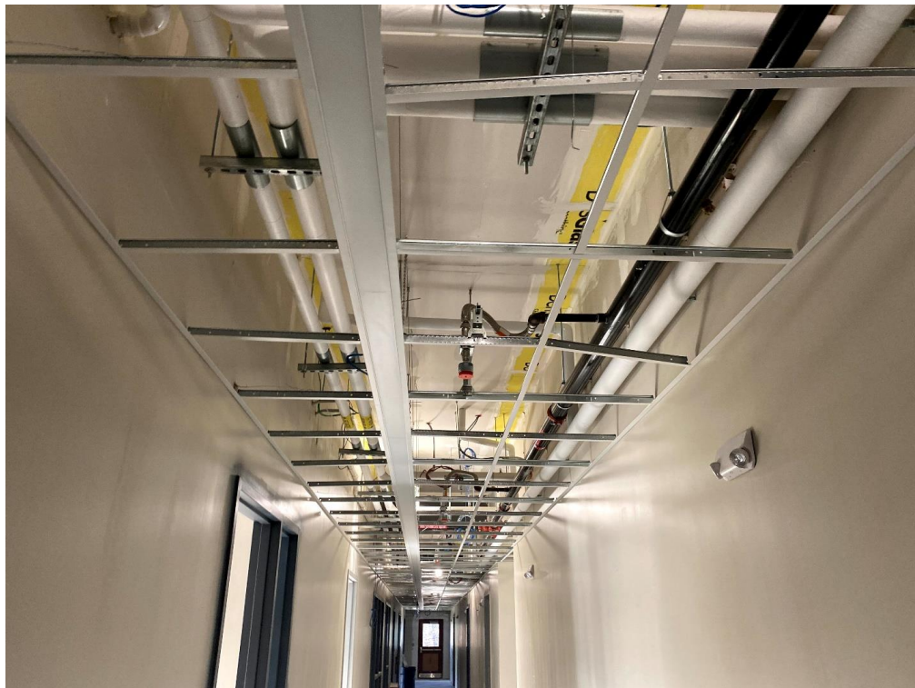
Ceiling Grid Completed
